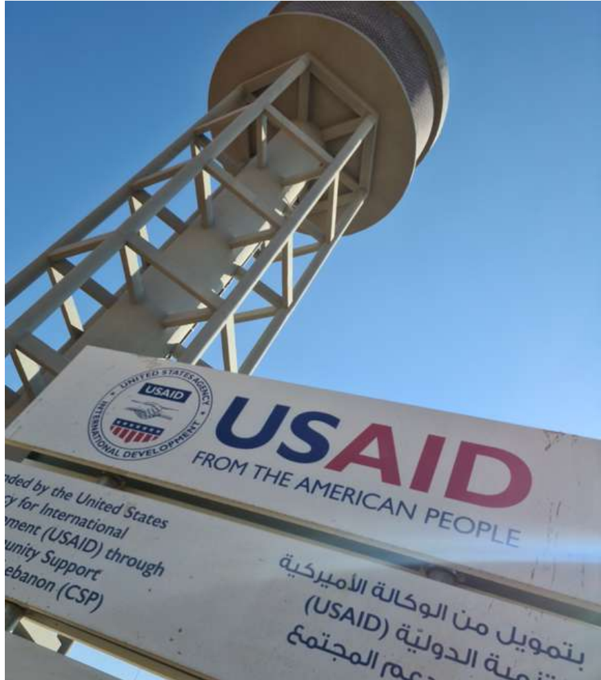
Completion of the 300m 3 elevated water tank in Talia
